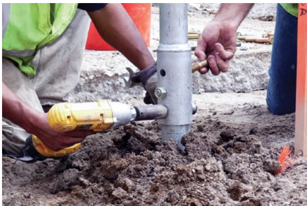
Figure 1.87 Install coupler bolts
