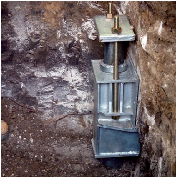
Figure 2.38 PP288 bracket ready for lift cylinder assembly
