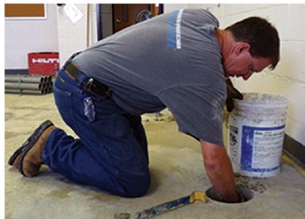
Figure 2.50 Excavating beneath the slab
