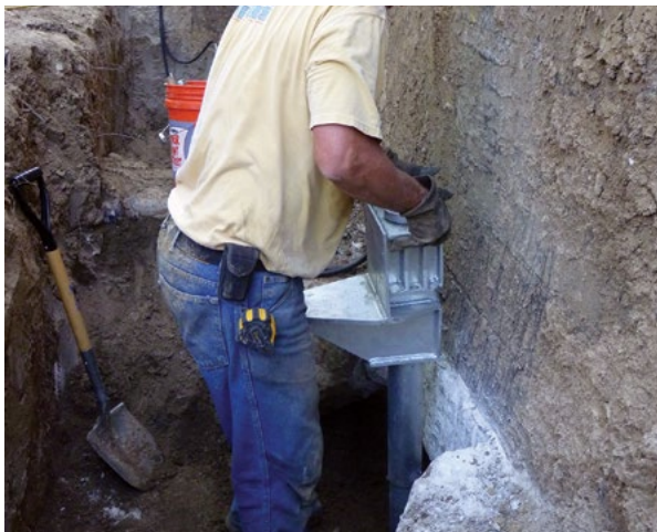
Figure 1.92 Lower assembly over pile shaft
