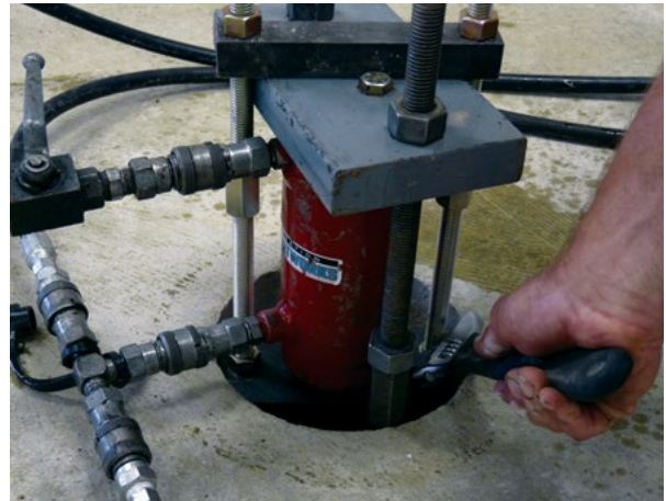
Figure 2.63 Pier load locked off by tightening nuts on top of pier cap
