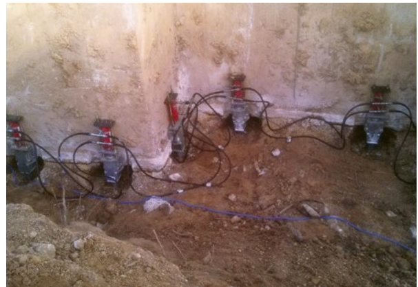
Figure 2.40 Hydraulic system connected to provide uniform application of load
