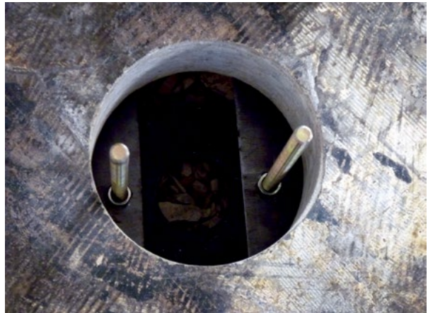
Figure 2.52 Threaded rods installed
