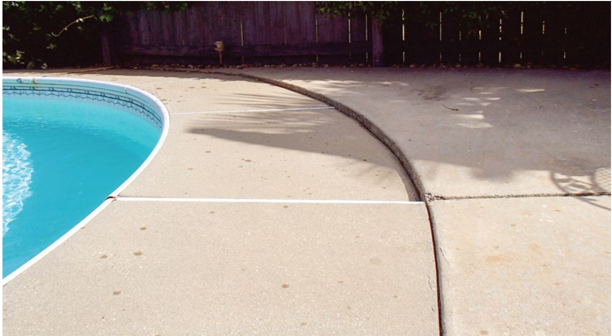
Figure 5.5 Pool deck slab settlement
