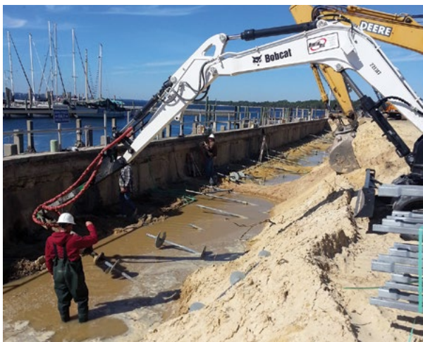
Figure 1.43 Helical tiebacks stabilize marina seawall
