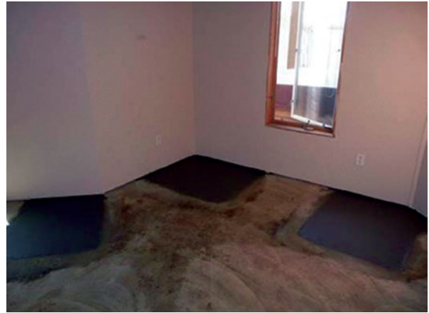
Figure 2.44 Concrete placement at interior pier locations
