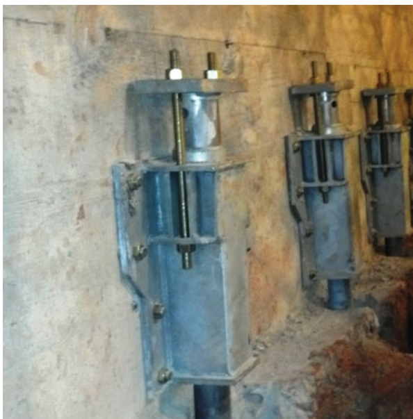
Figure 2.45 Flush-mount bracket installation
