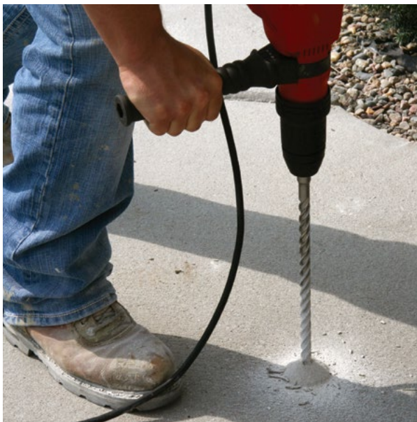
Figure 5.15 Concrete slab drilled to provide access holes
