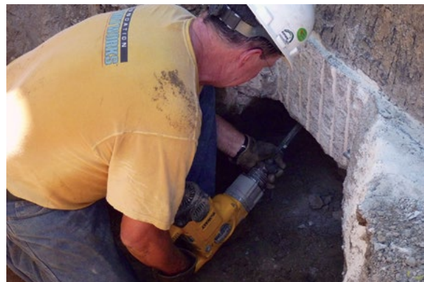
Figure 1.90 Footing preparation
