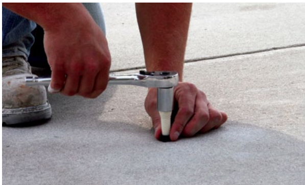
Figure 5.16 Injection port tightened with a socket wrench
