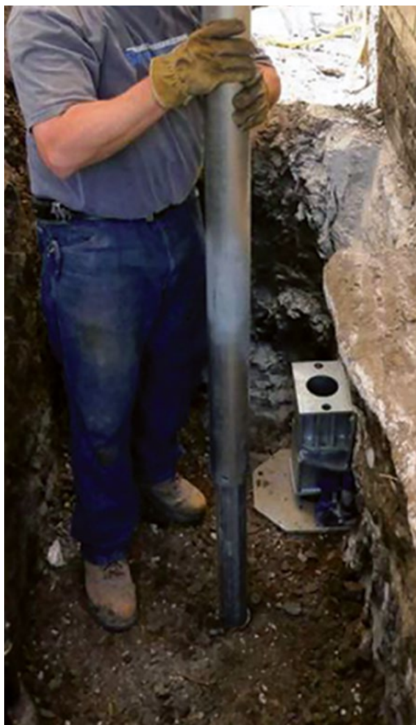
Figure 2.24 Exterior sleeve slid over the starter tube
