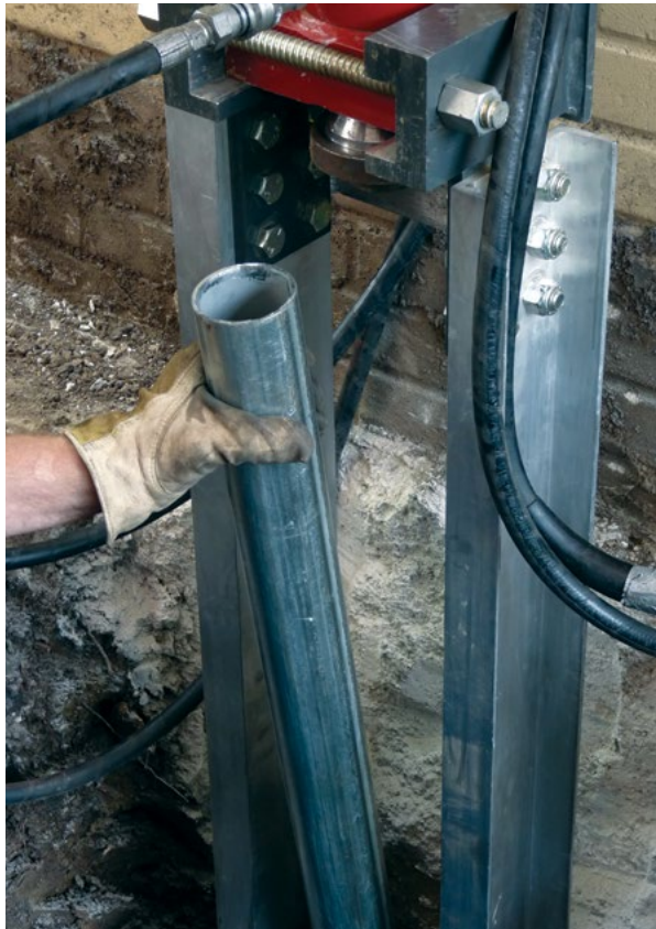
Figure 2.33 Installing PP288 push pier tube
