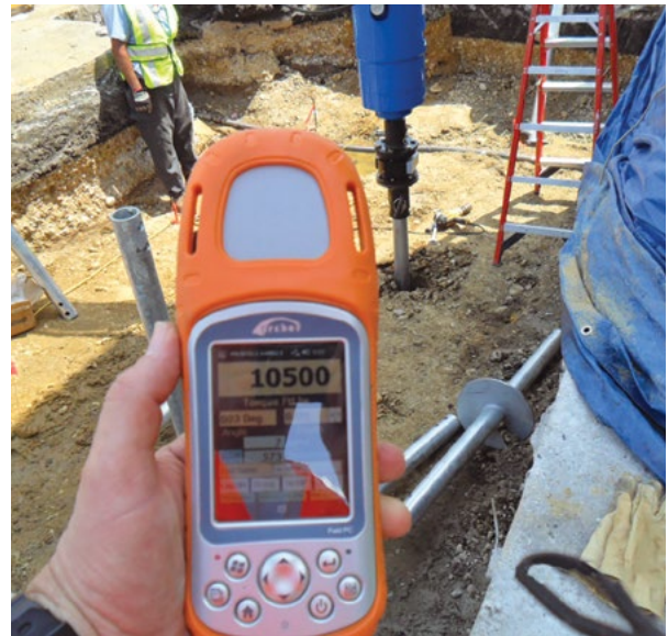
Figure 1.86 Torque transducer providing direct reading of torque for helical pile project at Reagan National Airport
