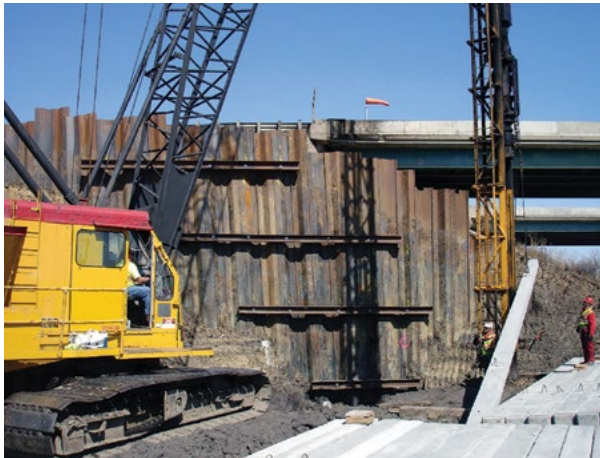
Figure 1.42 Multi-tier helical tieback installation to support sheet pile wall
