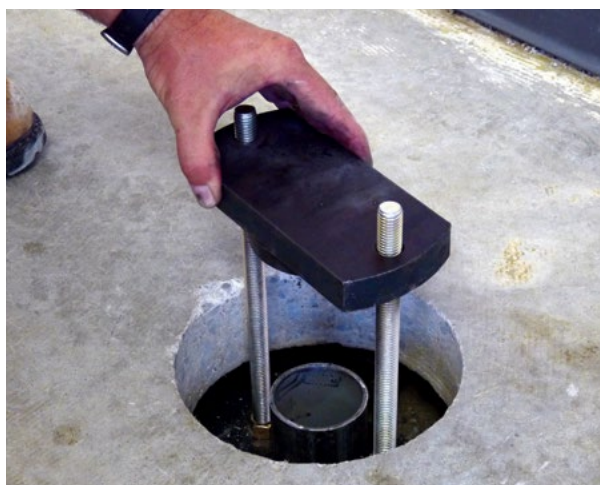
Figure 2.57 Pier tube cut to length; pier cap placed
