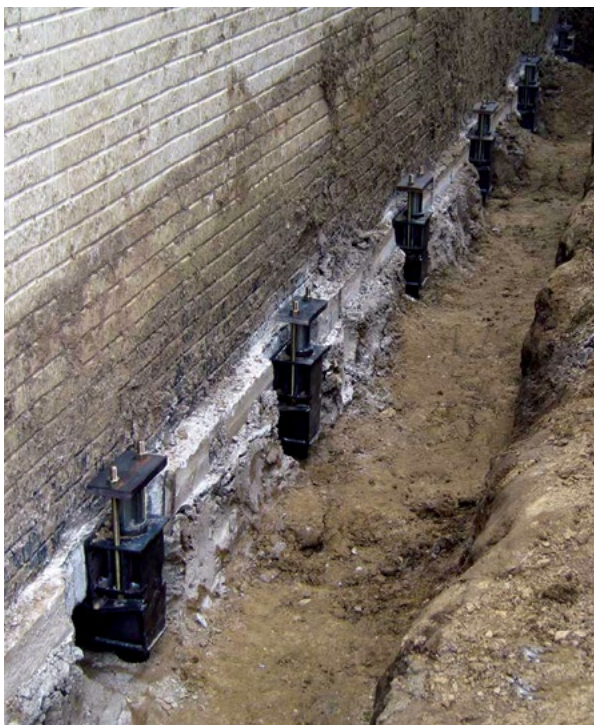
Figure 2.41 System locked off; pier installation complete
