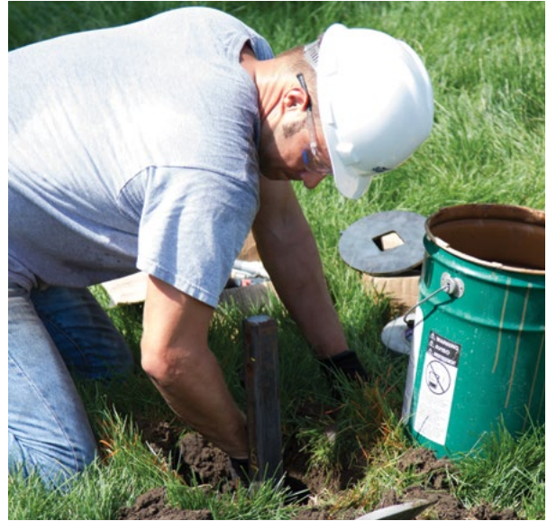
Figure 1.101 Excavating for the reservoir and removing loose soil
