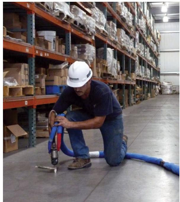
Figure 5.6 PolyLevel stabilizes warehouse floor slab
