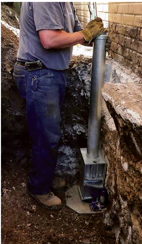
Figure 2.25 Sleeve and starter inserted together through the bracket
