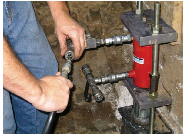
Figure 2.39 Connection of lift cylinder assembly
