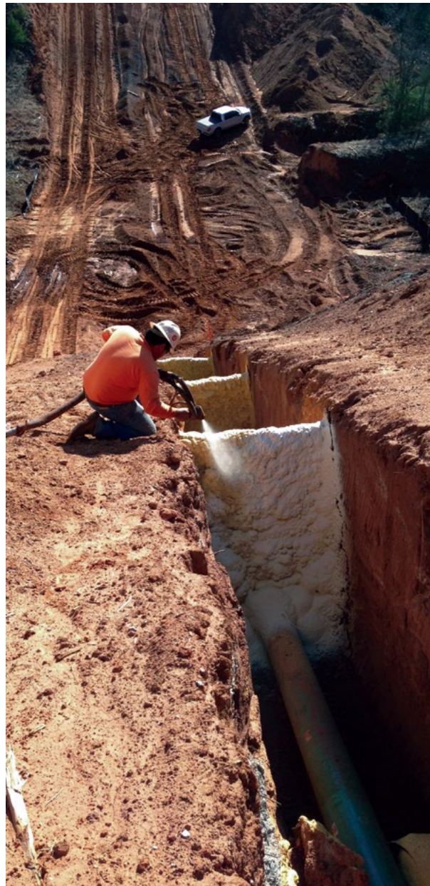
Figure 5.10 Placement of polyurethane foam trench breaks
