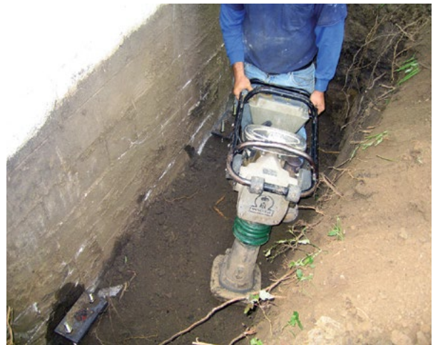
Figure 1.96 Backfill and compact soil
