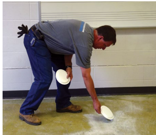
Figure 2.46 Marking slab pier locations
