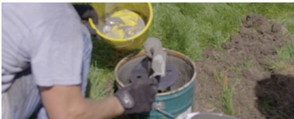
Figure 1.106 Buttering the top of pile at coupler
