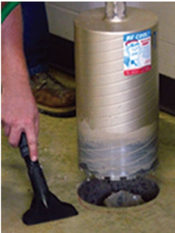
Figure 2.48 Concrete coring
