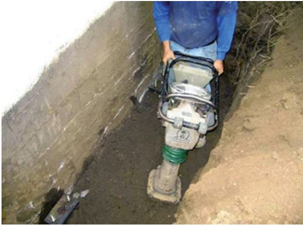
Figure 2.43 Backfill excavations and compact soil
