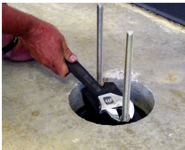
Figure 2.58 Lightly tighten pier cap down onto pier tube
