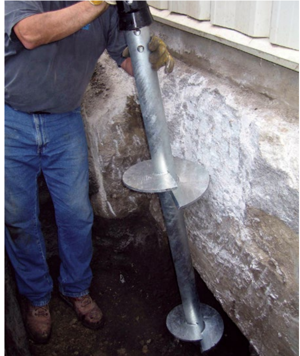
Figure 1.91 Alignment of lead
