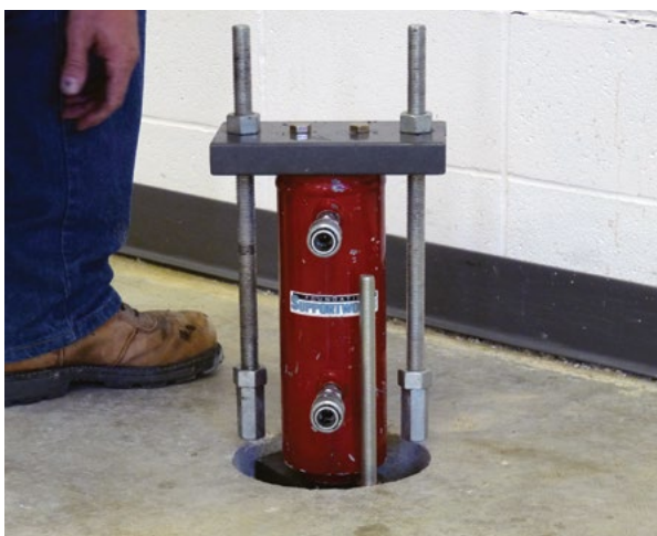
Figure 2.59 Lift cylinder assembly set on pier cap
