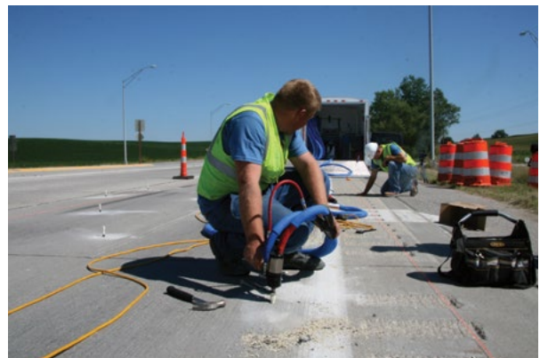
Figure 5.12 Monitoring pavement lift with string lines
