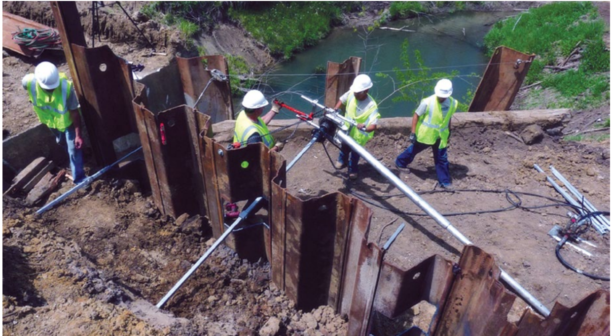
Figure 1.5 Helical tieback installation with hand-held equipment
