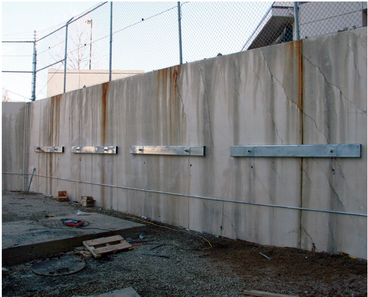
Figure 1.45 Helical tiebacks and tube steel walers stabilize concrete retaining wall
