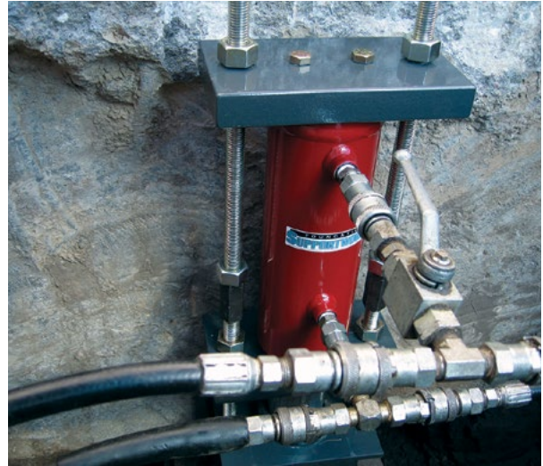
Figure 1.95 Set hydraulic lift cylinders
