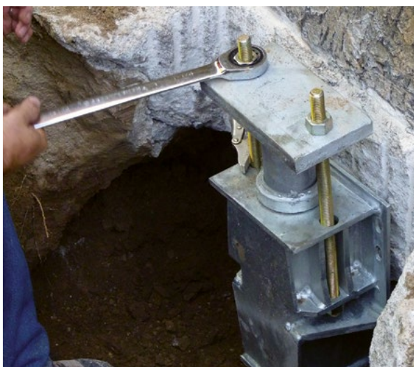
Figure 1.94 Install cap plate and rods
