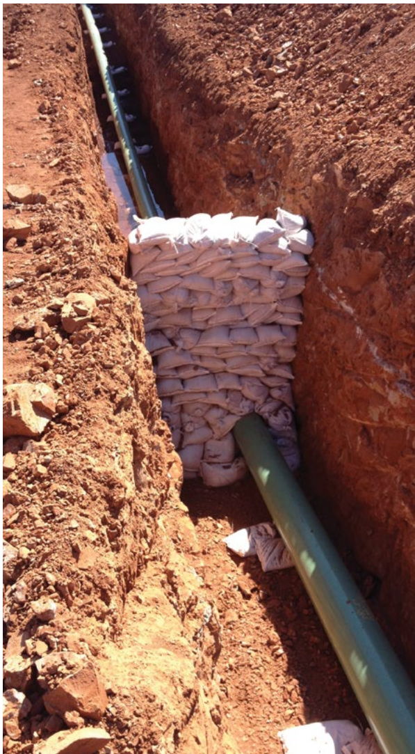
Figure 5.9 Sandbag trench breaker for pipeline
