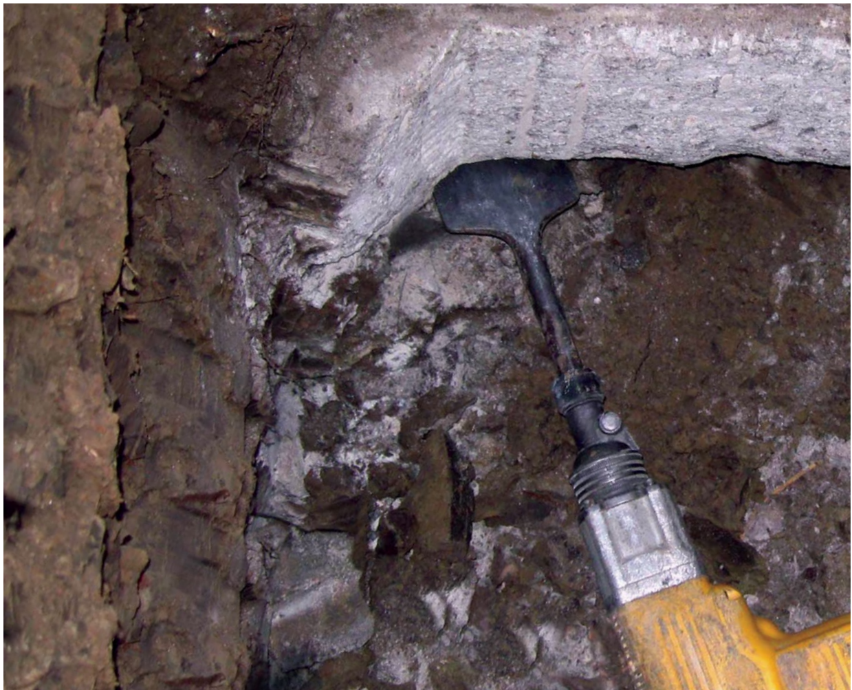
Figure 2.18 Removing soil from beneath the footing with a chisel attachment
