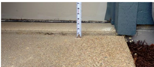
Figure 5.4 After: Driveway lifted back to near original elevation
