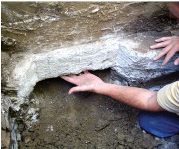
Figure 2.20 Checking underside of footing for proper preparation
