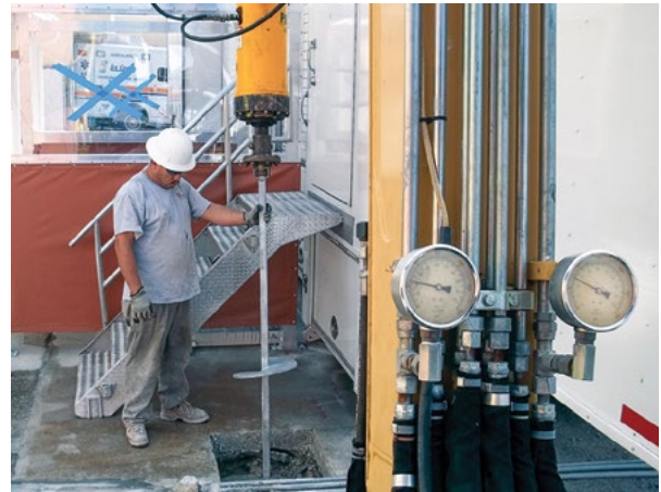
Figure 1.81 Monitoring pressure gauges while installing square shaft helical anchor
