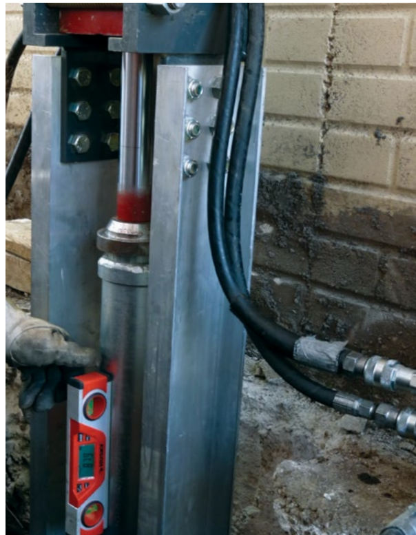
Figure 2.31 Checking drive stand alignment with digital level
