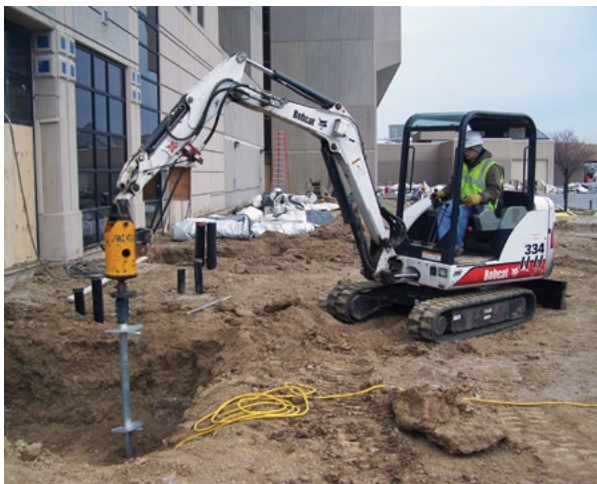
Figure 1.3 New construction helical pile installation
