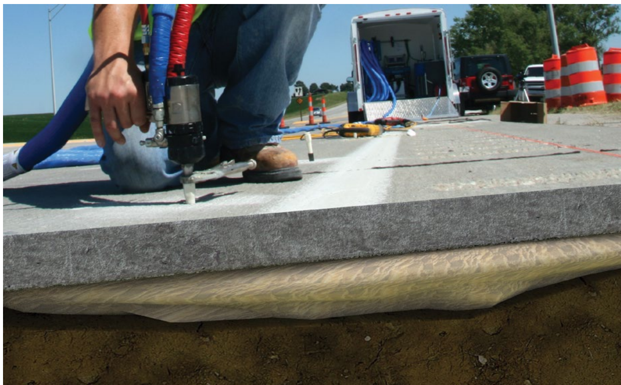
Figure 5.1 Rendering of PolyLevel foam injection beneath concrete pavement
