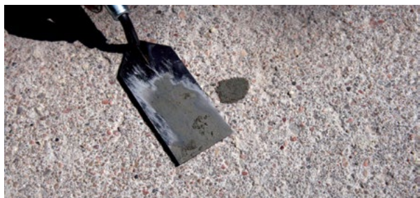
Figure 5.18 Patching the injection hole
