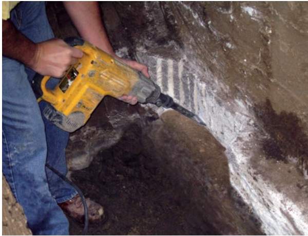
Figure 2.19 Smoothing the vertical and horizontal bearing surfaces with a chipping hammer
