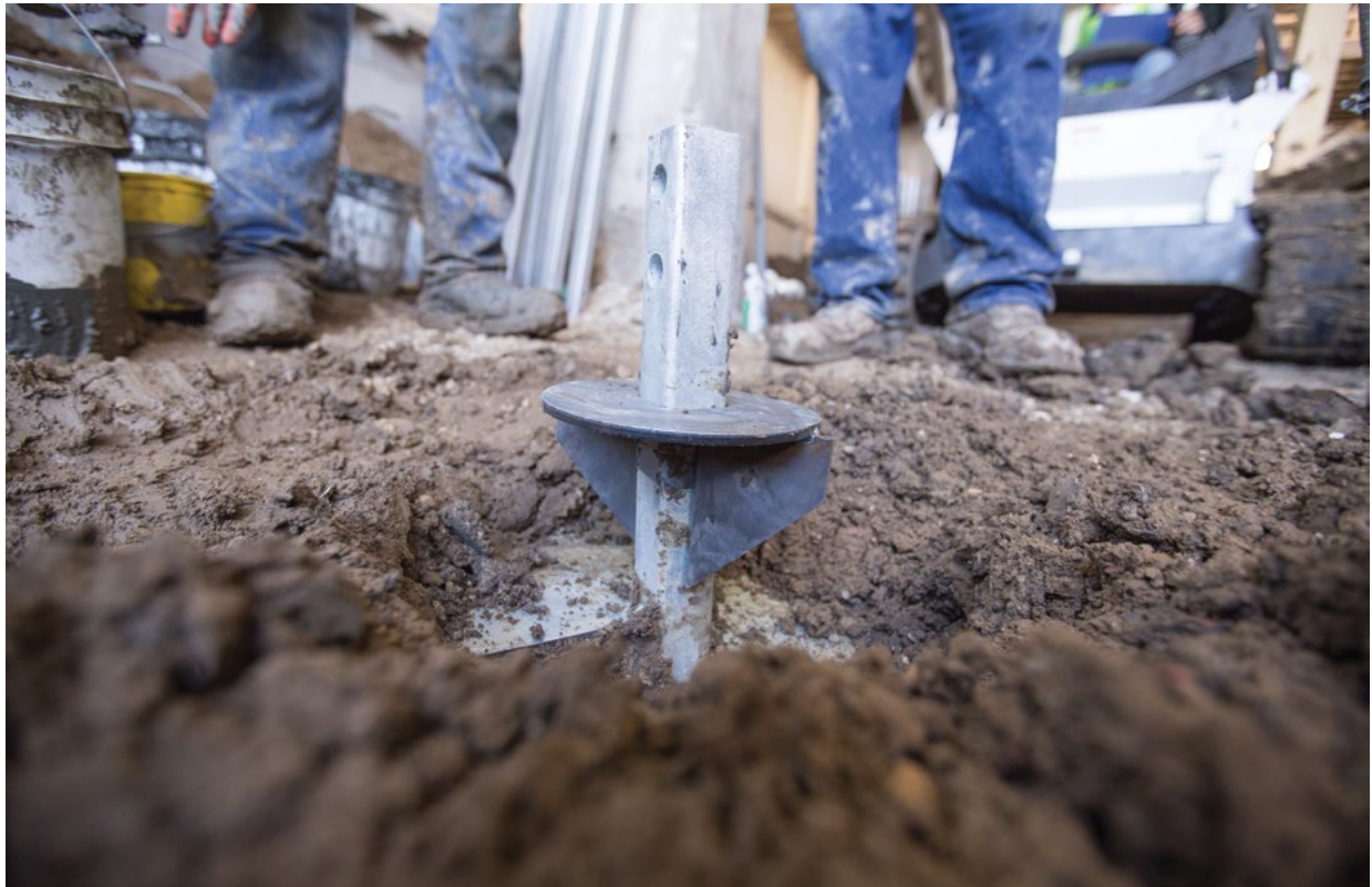
Figure 1.59 Spiked Lead Displacement Plate
