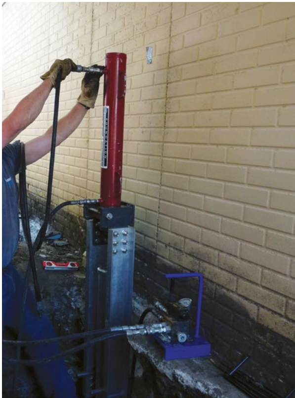
Figure 2.30 Connect hydraulic hoses
