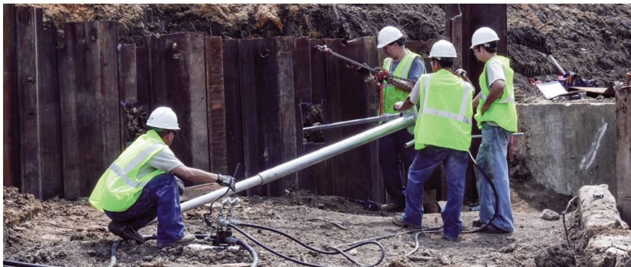
Figure 1.76 Torque arm
