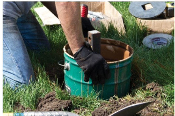
Figure 1.102 Setting the reservoir
