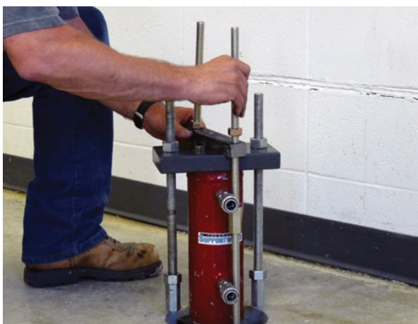
Figure 2.60 Lift plate assembly coupled to threaded rods of slab pier bracket
