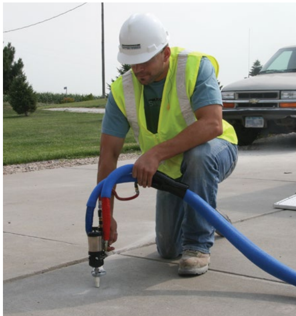
Figure 5.17 PolyLevel foam injected below the slab
