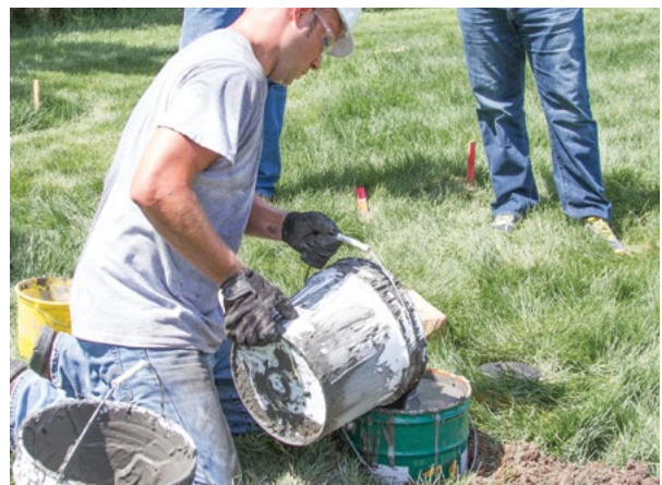
Figure 1.103 Pouring grout into the reservoir
