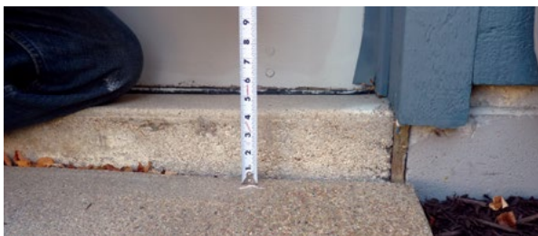
Figure 5.3 Before: Driveway settled up to 4 inches relative to garage slab
