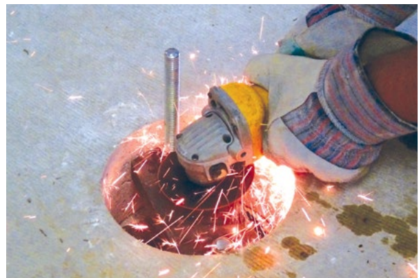
Figure 2.64 Cutting the threaded rods
