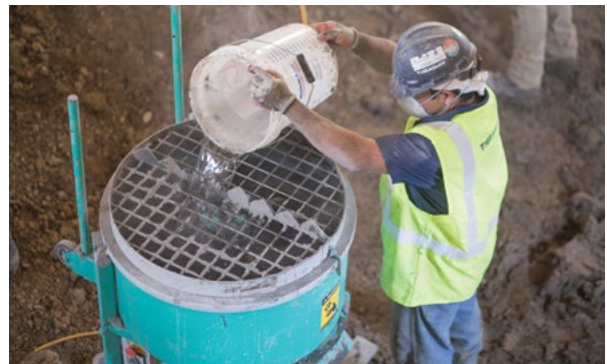
Figure 1.98 Grout mixing
