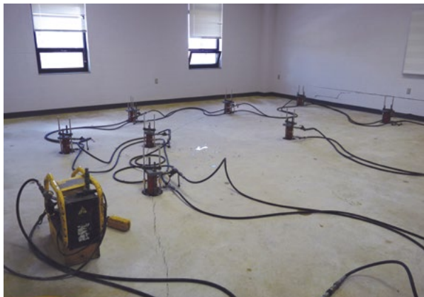
Figure 2.62 Lift cylinders connected for simultaneous loading
