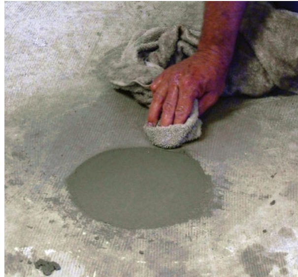
Figure 2.66 Finishing concrete
