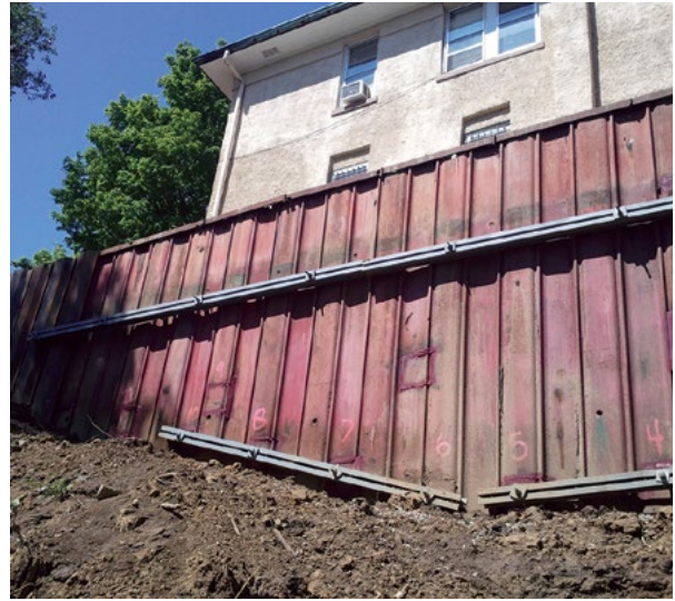
Figure 1.44 Helical tiebacks stabilize sheet pile wall below historic home
