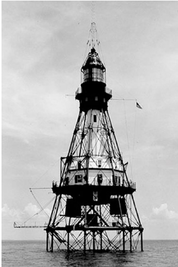
Figure 1.1 Lighthouse supported by screw (helical) pile foundations
