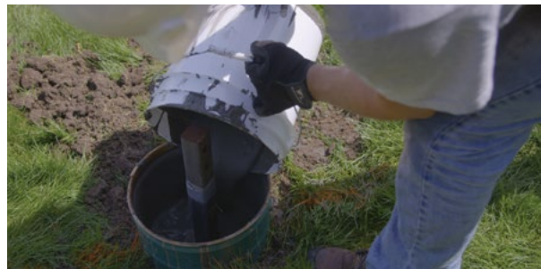
Figure 1.108 Maintaining an adequate level of grout within the reservoir
