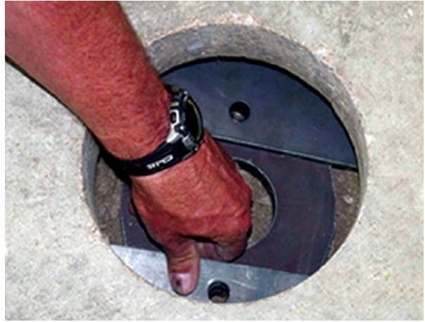
Figure 2.51 Main plate and wing plates positioned and aligned beneath the slab
