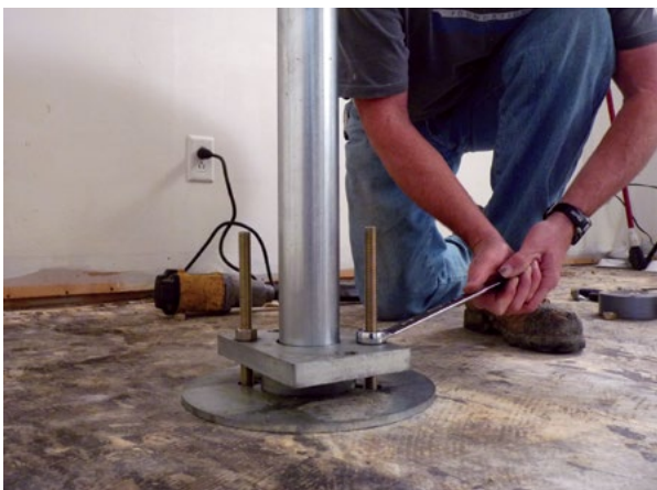
Figure 2.54 Slab pier drive adaptor installed
