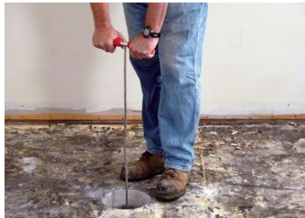
Figure 2.49 Probing for utilities or obstructions
