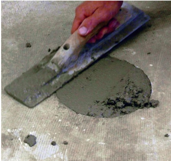
Figure 2.65 Patching holes at pier locations
