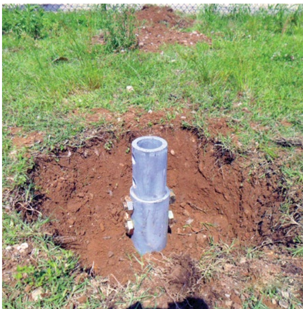
Figure 1.12 Internal detached coupler detail of HP450
