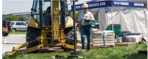
Figure 1.97 Grout mixing station near work area
