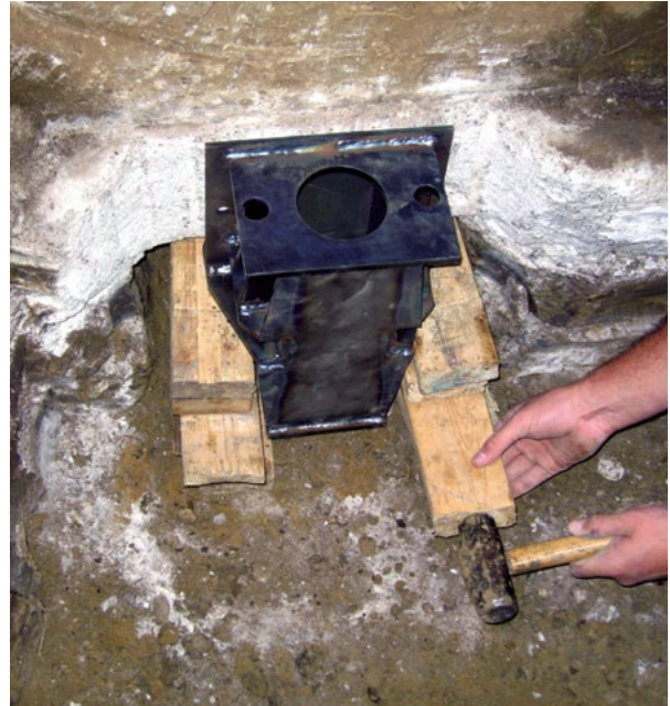
Figure 2.22 Temporary bracket support with wood cribbing
