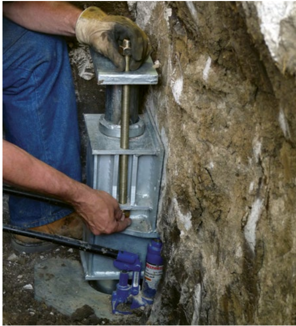
Figure 2.37 Installation of pier cap plate with threaded rods and nuts
