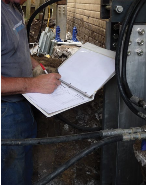
Figure 2.35 Pressure readings are recorded for each pier tube
